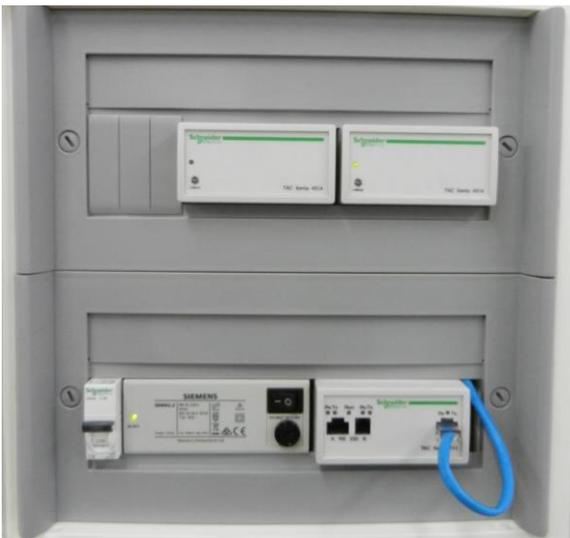
Fig. 6. Controller Xenta 711 connected with 2 I/O boards Xenta 451A.
