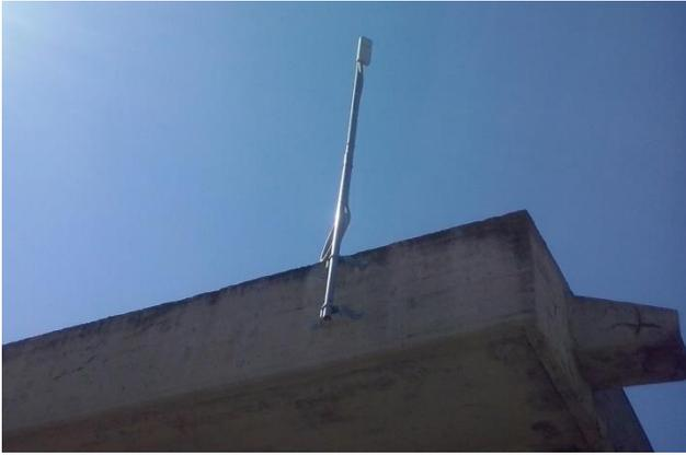
Fig. 5. 5GHz Wi-Fi Transmitter
