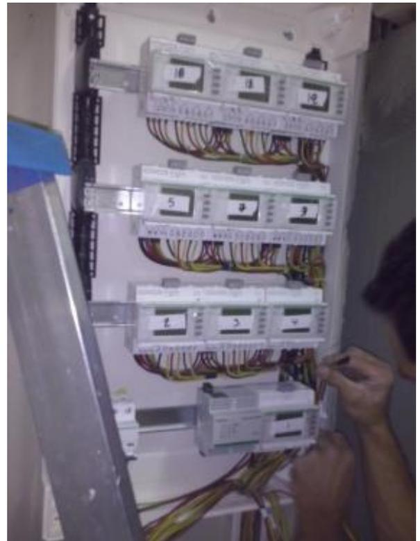
Fig. 4. Installation of 10 Meters PM3250 and 1 Gateway EGX100 at building M of Mechanical Engineer faculty
